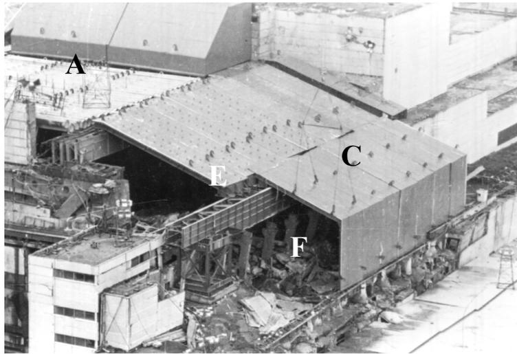
*FIG. 6.5. Major structural components of the Chernobyl Shelter: (A) pipe roofing, (B) southern panels, (C) southern hockey sticks, (D) B1/B2 beams, (E) mammoth beam, and (F) octopus beam.*
