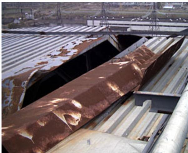
FIG. 6.3. Opening at the “Shelter” allowing infiltration of atmospheric water.
